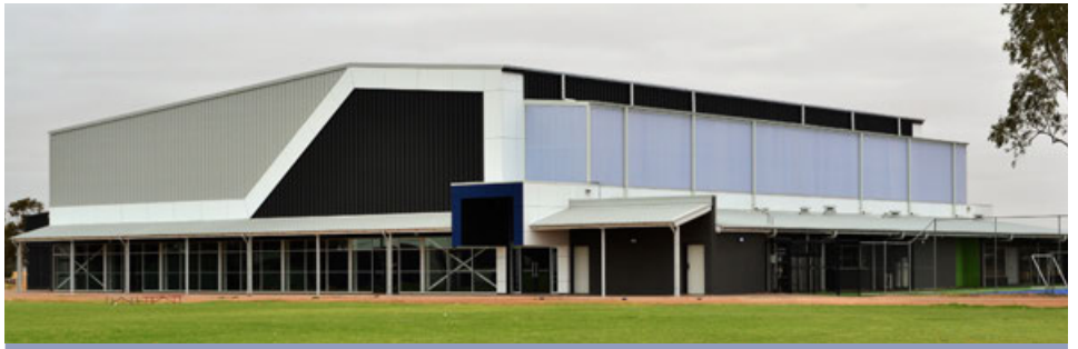
SPORTS CENTRE: The St Mark's Sports Centre is finished and open! Our students are flourishing in the amazing new facility which includes a double court gymnasium.
